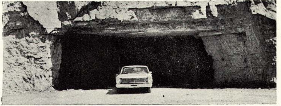
A NEW FORD CUSTOM in the entrance of the Ford storage area shows the size. This entrance has been sealed off, an overhead door hung and an unloading well for trucks dug out. The unloading facility will accommodate two huge vans at a time.
